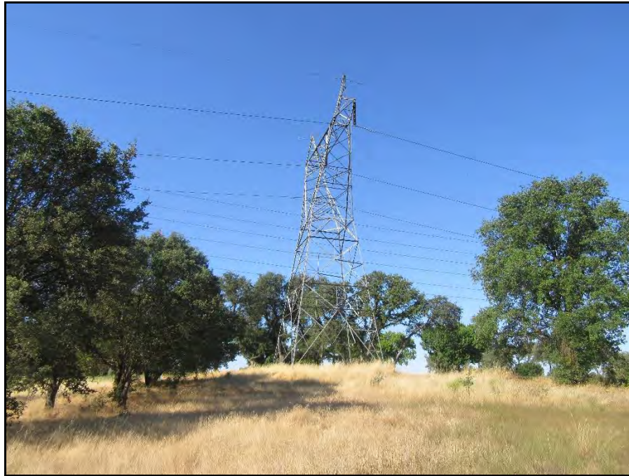
P-31-3280 transmission tower (view south; June 23, 2020).
